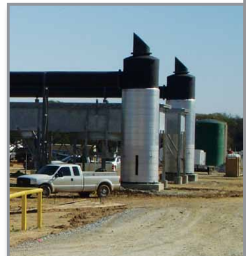
Ground Access Installation
